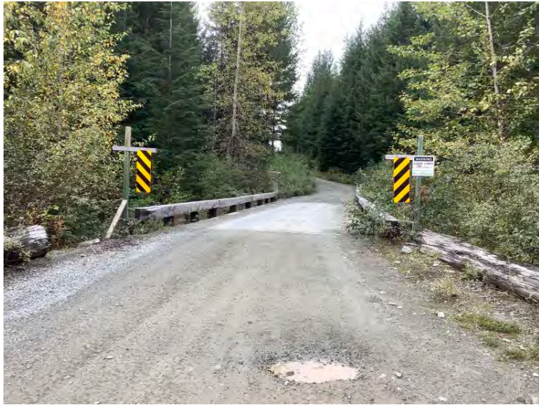
Approach from Right Bank when facing downstream
