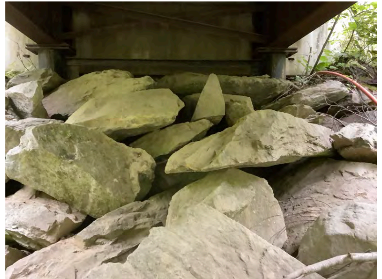
Right Bank Abutment when facing downstream
