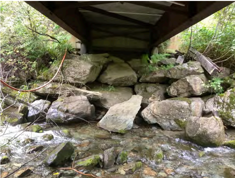
Left Bank Abutment when facing downstream
